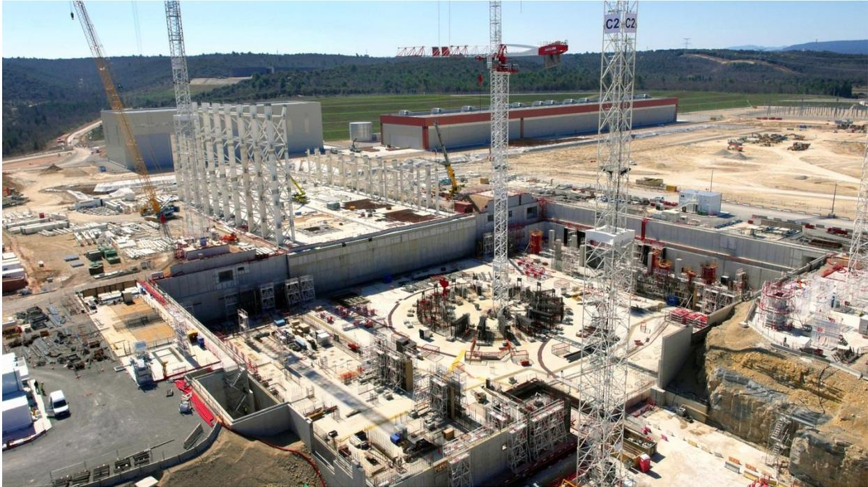
**Figure 1.** Construction site for the \$16 billion ITER located in Cadarache, France (near Monaco) that is sponsored by seven participants; the European Union, India, Japan, China, Russia, South Korea, and the United States. The circular structure in the center-right is the footing for a 500 Megawatt hot fusion plasma reactor that is projected to become operational around 2027.
